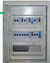
House Electric Fuse Box
